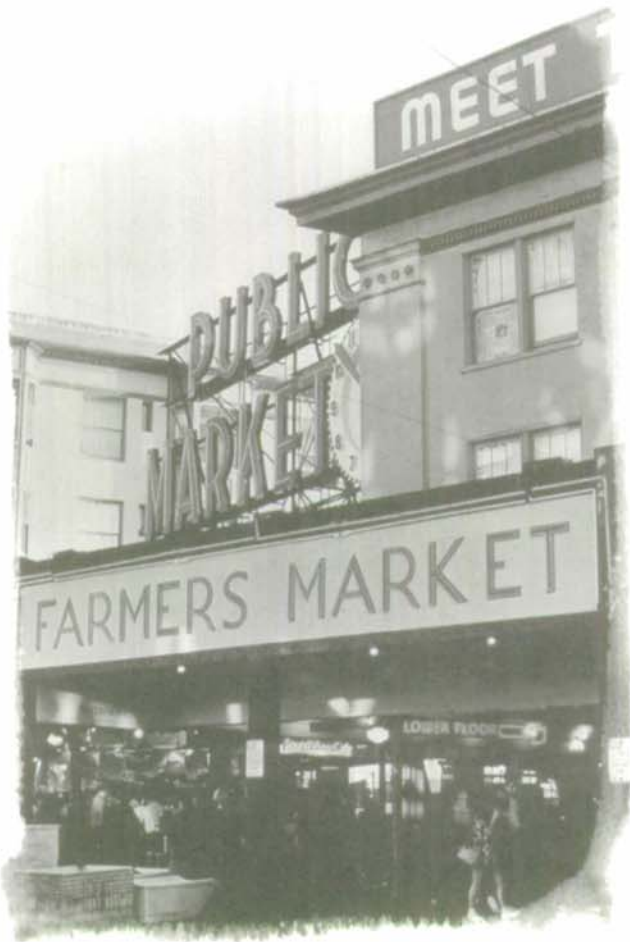
Historic cobblestone streets lead to Seattle's Pike Place Market, one of the last remaining working farmer's markets in the country. Photo courtesy of the Seattle-King County Convention & Visitors Bureau.
