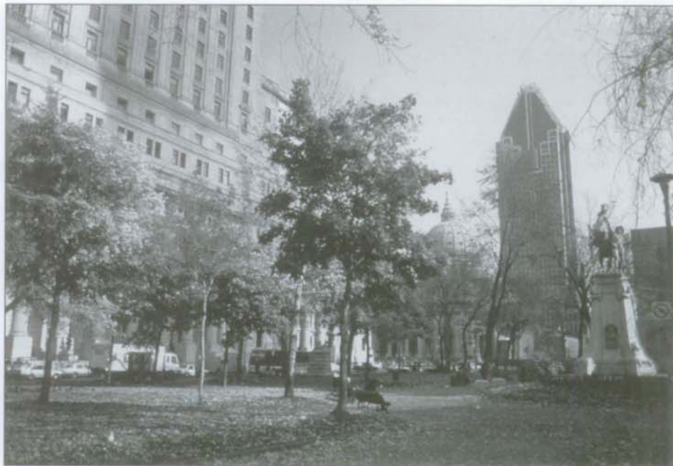
Dorchester Square (Sun Life and 1000 de La Gauchetière buildings) - downtown • Courtesy of Greater Montréal Convention and Tourism Bureau
