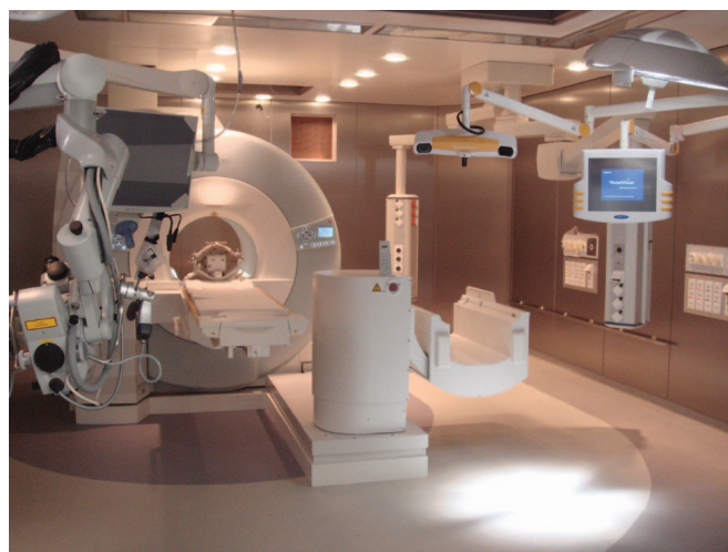
FIGURE 17.2. INI-Brain-Suite with a 1.5-T MRI scanner. Note the head fixation with the coil in the gantry and the console for the rotating table in front. On the right is a ceiling-mounted infrared camera and touch screen of the navigation system. On the left is a multivision navigation microscope. The curved line on the floor (right front corner) indicates the 5-G line.
