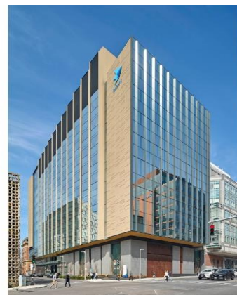
Klarman building - 350,000-square-foot, 10-story – opened 2023
